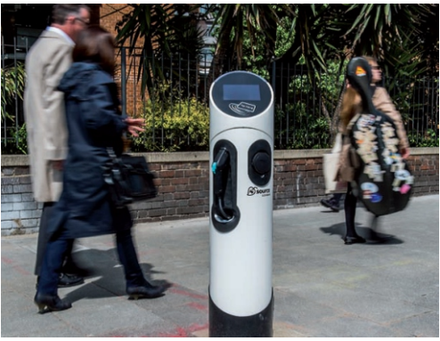
7kW charge point post
